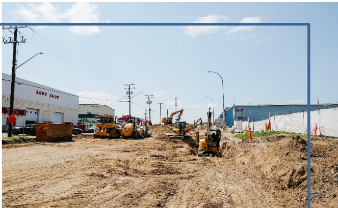
York Road Reconstruction
