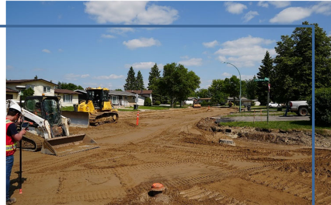
Circlebrooke Water Main Replacement
