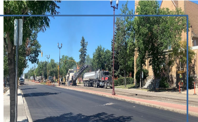
Smith Street Paving
